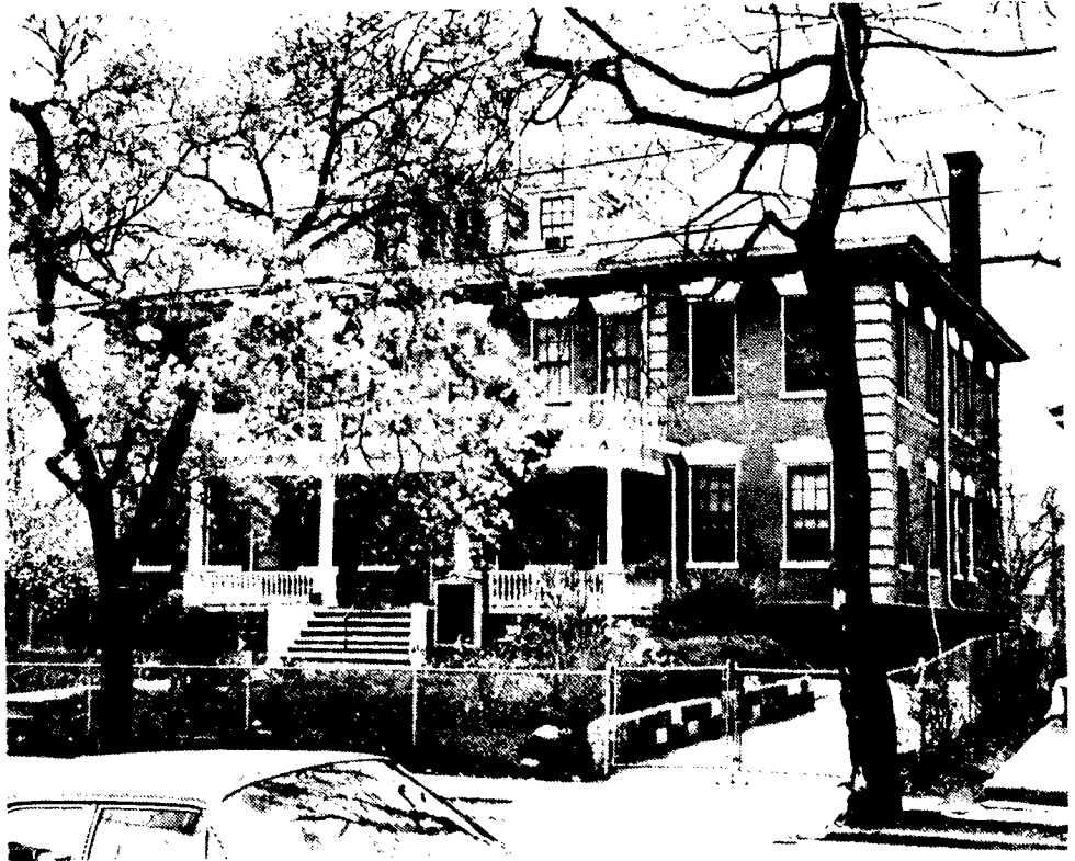
Church property at 22 Halleck Street in North Newark provides a comfortable Church home and chapel for the members.
